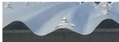
Serrage excessif
