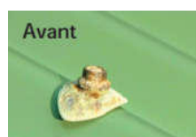
Serrage excessif
