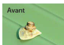
Serrage excessif
